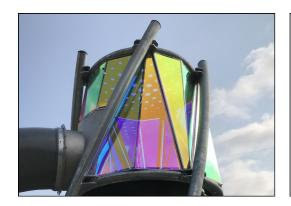
The graphic panels are made of high-quality polycarbonate with a thickness of 6mm. The color changing dichroic film is glued on the outside. The PC panels are UV stabilized to prevent degradation.
