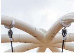
Corocord aluminium clamps are used as connectors between steel posts and rope. The aluminium casting is screwed into the steel post and connects safely to the rope.
