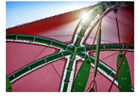
As an option, sunshading can be integrated into the Giant Dome. The lightweight, durable and semitransparent tissue perfectly complements the colourful design, while blocking up to 79% of solar radiation and protecting the children.
