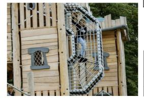
The wire frame tunnel is made of hot dip galvanized high quality steel. Corocord 16mm ropes are special 'Hercules'-type with galvanized four-stranded steel wires and a steel wire core. Each strand is tightly wrapped with PES yarn, which is melted onto each individual strand.
