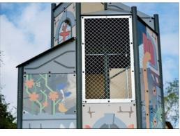
Fully welded steel frame with 45° cross welded steel grid of round steel pins with a diameter of 4mm. The airflow panel contributes to the overall structural integrity of the GIANT towers.
