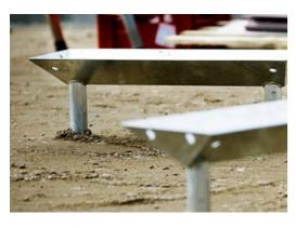
The cubes are supported by a unique designed footing system that secures the correct positioning of the cubes.
