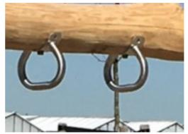
Overhead climbing handles are made of high quality stainless steel. The handles are attached to the upper robinia crossbeam by stainless steel hardware.
