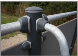
The connectors are made of die-cast aluminium.
