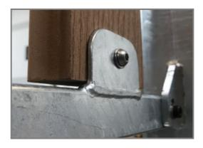
The WPC boards are attached to  $70 \times 45 \times 3$ mm welded flanges with stainless steel M8 bolts, nuts and washers. These connections are not visible from the inside and create a safe and robust connection.
