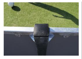
The posts are made of 80 x 80 x 3mm profile with horizontally, 6mm welded flanges. This will enable easy installation and strong construction. The low-density polyethylene post caps are attached with blind rivets.
