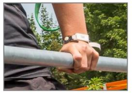
The bars intended for exercises are made of hot-dip galvanised steel ø48mm. The diameter of these bars provide a good support when used to for push ups exercises or when doing exercises standing on the tubes.
