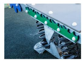
The usage of two springs and a center tipping point makes possible for users of different ages to play together. The tipping point bushing is a made of high quality nylon (PA6).
