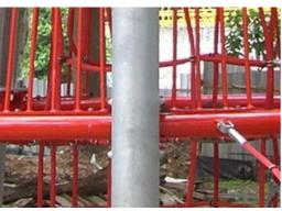
The metal parts are made from high-quality steel consisting of hot-dip galvanisation on both the inside and outside and also includes leadfree zinc and an additional layer of powder coating. This ensures both excellent corrosion resistance and colourful design expression.
