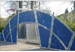
The goal measures ~140cm in depth and ~330cm in width, with all posts made of galvanized steel with a hot dip galvanized surface treatment. The front frame is made with Ø48 tubing, and the backside of the goal uses ten tubes with a diameter of Ø38.
