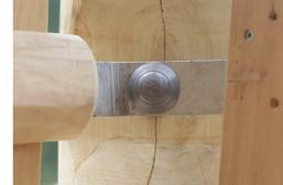
The hardware is made of stainless steel or galvanised steel to ensure durable connections with a high corrosion resistance.
