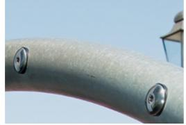
The steel arches are hot dip galvanised inside and outside with lead free zinc. The galvanisation has excellent corrosion resistance in outside environments and requires low maintenance. Corocord aluminium clamps are used as connectors between steel posts and rope. Two aluminium castings are bolted together. The height of the clamps is thus variable.
