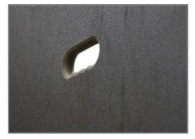
The wall surface is made of 17.8mm thick High Pressure Laminate (HPL) panels to ensure optimal strength and durability.
