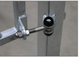
The hinges on the entrance gate are 16mm and made of Stainless Steel, the handle can be accessed from both inside and outside of the pitch but is constructed in such a way that it remains fully flat on the inside of the MUGA.
