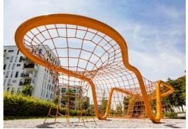
The steel surface of these bended steel pipes are wet painted with one basic layer and one top layer of lead free color material. The paint has excellent corrosion resistance and can be easily maintained.
