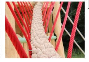
Corocord ropes of the bridge are special 'Hercules'-type with galvanised six-stranded steel wires and a steel wire core. The PP rope in coconut style has a diameter of 15 cm. The internal steel wire core has thimbles at both ends, which serve as attachments for the rope to existing connecting elements.
