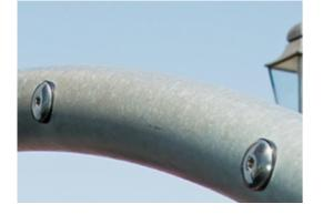
The steel structure are hot dip galvanised inside and outside with lead free zinc. The galvanisation has excellent corrosion resistance in outside environments and requires low maintenance.
