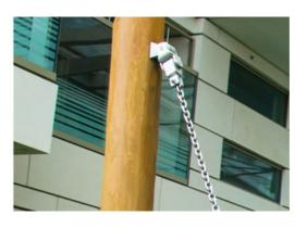
Swing suspensions are made of polyamide and consist of double ball bearing system with swivel.
