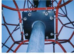
Corocord membranes consist of friction-proof rubberized material of conveyor belt quality with excellent UV resistance. Tested and compliant with REACH requirements for PAH. Embedded is a four-layered armoring made of woven polyester. The armoring and the two surface layers result in a total thickness of 7.5 mm.
