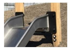
Slide interface panel of 19mm EcoCore™ which a highly durable, eco-friendly material, which is not only recyclable after use, but also consists of a core produced from 100% recycled material.
