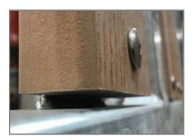
The Wood Plastic Composite panels are made of 100% recycled fibre/wood powder and High Density Poly Ethylene (HDPE). With the dimensions of 860 x 110 x 30mm the boards are extremely strong.
