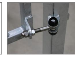
The hinges on the entrance gate are 16mm and made of Stainless Steel, the handle can be accessed from both inside and outside of the pitch but is constructed in such a way that it remains fully flat on the inside of the MUGA.
