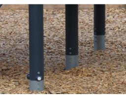
Main posts with hot dip galvanized steel footing are available in different materials: Pressure impregnated pine wood posts. Pre-galvanized inside and outside with powder coated top finish steel posts. Lead free aluminium with color anodized top finish.
