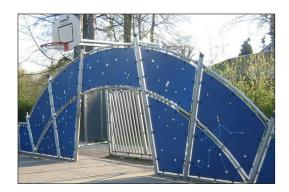
The goal measures ~140cm in depth and ~330cm in width with all posts made of galvanised steel with a hot dip galvanised surface treatment. The front frame is made with Ø48 tubing, and the backside of the goal uses 10 tubes with a diameter of ø38
