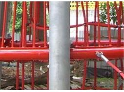
The metal parts are made of high quality steel, hot dip galvanised inside and outside with leadfree zinc. On the outside, there is an additional layer of powder coating. This ensures both excellent corrosion resistance and colourful design expression.
