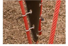
Corocord membranes consist of friction-proof rubberized material of conveyor belt quality with excellent UV resistance. Tested and compliant with REACH requirements for PAH. Embedded is a four-layered armoring made of woven polyester. The armoring and the two surface layers result in a total thickness of 8mm.
