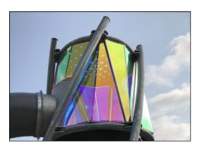
The graphic panels are made of high-quality polycarbonate with a thickness of 6mm. The color changing dichroic film is glued on the outside. The PC panels are UV stabilized to prevent degradation.
