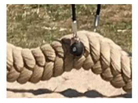
The chain/ropes are attached to the Coconut rope by KOMPAN swivel bushings made of stainless steel with bronze bearings. The swivels have an outside cover of black PUR. The usage of side mounted swivels provides frictionless movement, eliminates fingers and feet entrapments and enlarges the standing surface on top of the rope.
