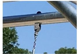
Unique designed swing hangers of stainless steel with anti-twist function. The hangers are attached to the cross beam by a bolt through connection to ensure high durability.
