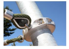
Corocord aluminium clamps are used as connectors between steel posts and rope. Two aluminium castings are bolted together. The height of the clamps is thus variable.
