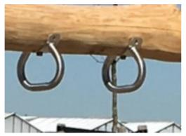
Overhead climbing handles are made of high quality stainless steel. The handles are attached to the upper robinia crossbeam by stainless steel hardware.
