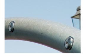
The steel structure are hot dip galvanized inside and outside with lead free zinc. The galvanization has excellent corrosion resistance in outside environments and requires low maintenance.
