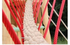
Corocord ropes of the bridge are special 'Hercules'-type with galvanised six-stranded steel wires and a steel wire core. The PP rope in coconut style has a diameter of 15 cm. The internal steel wire core has thimbles at both ends, which serve as attachments for the rope to existing connecting elements.
