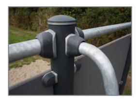
The connectors are made of die-cast aluminium, specially alloyed for the outdoor environments and heavy usage. The screws attaching the connectors are stainless steel and protected by zinc washers.
