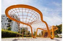
The steel surface of these bent steel pipes are painted with one basic layer and one top layer of lead-free colour material. The paint has excellent corrosion resistance and can be easily maintained.
