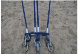
Huge spacenet structures are secured to the foundation with a system of three turnbuckles. Horizontal and vertical edge cables are fixed to individual turnbuckels, wich then connect to individual steel anchors. This system ensures that each edge cable can be tensioned separately and increases strucutral safety by way of independent anchoring.
