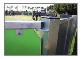
The HDPE panels are connected with M8 stainless steel bolts to 42.5 x 40 x 3mm welded flanges. These connections are not visible from the inside and create a strong and safe connection.
