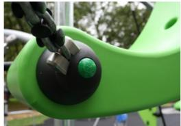
More substantial play activities are made of 100% recyclable PE. The play shell displayed is moulded in one piece with a minimum 5mm wall thickness. PE has high impact resistance across a wide temperature span which ensures vandal resistance in all locations.
