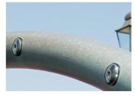
The steel structures are hot-dip galvanised inside and outside with lead free zinc. The galvanisation has excellent corrosion resistance and requires low maintenance.
