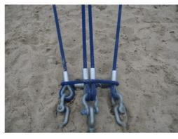
Huge spacenet structures are secured to the foundation with a system of three turnbuckles. Horizontal and vertical edge cables are fixed to individual turnbuckels, wich then connect to individual steel anchors. This system ensures that each edge cable can be tensioned separately and increases strucutral safety by way of independent anchoring.
