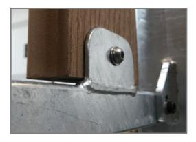
The WPC boards are attached to  $70 \times 45 \times 3$ mm welded flanges with stainless steel M8 bolts, nuts and washers. These connections are not visible from the inside and create a strong and safe connection.
