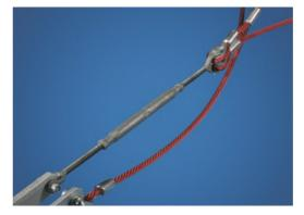
The spacenets' main bearing ropes are equipped with an additional safety feature: should the main connections fail, the safety rope prevents collapse of the structure.
