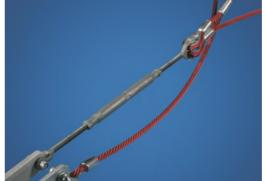
The spacenets' main bearing ropes are equipped with an additional safety feature: should the main connections fail, the safety rope prevents collapse of the structure.
