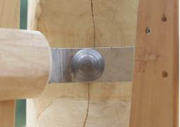
The hardware is made of stainless steel or galvanised steel to ensure durable connections with a high corrosion resistance.
