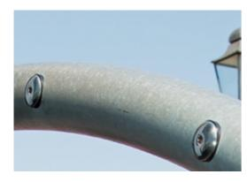
The steel structure are hot dip galvanised inside and outside with lead free zinc. The galvanisation has excellent corrosion resistance in outside environments and requires low maintenance.
