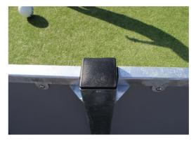
The posts are made of  $80 \times 80 \times 3$ mm profile with horizontally, 6mm welded flanges. This will enable an easy installation and strong construction. The low-density polyethylene post caps are attached with blind rivets.
