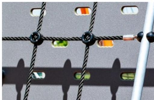
The ropes are made of UV-stabilised PES with inner steel cable reinforcement. The rope is induction treated in order to create a strong connection between steel and rope which leads to good wear resistance.
