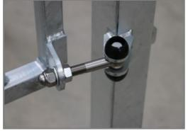
The hinges on the entrance gate are 16mm and made of Stainless Steel, the handle can be accessed from both inside and outside of the pitch but is constructed in such a way that it remains fully flat on the inside of the MUGA.
