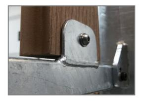
The WPC boards are attached to 70 x 45 x 3mm welded flanges with stainless steel M8 bolts, nuts and washers. These connections are not visible from the inside and create a strong and safe connection.
